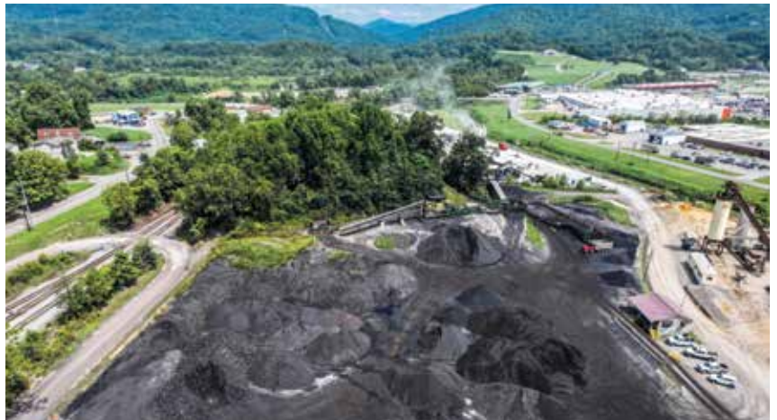
Located in Middlesboro, Ky., Premium Processing Company Inc. provides coal processing services.
